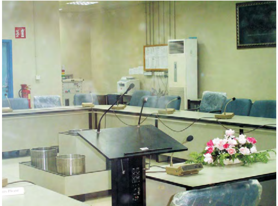
View of ECC Room and Communication Facility at ECC.
