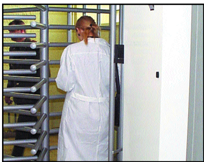
An access control system, including a nuclear materials portal monitor and turnstile prevents entry of unauthorized personnel.
