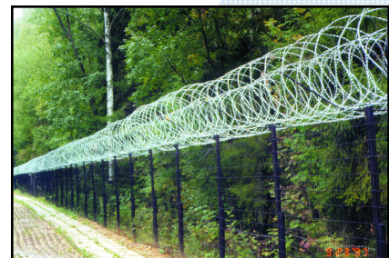
An upgraded perimeter with improved fence, clear zone, and intrusion detectors provide increased security.
