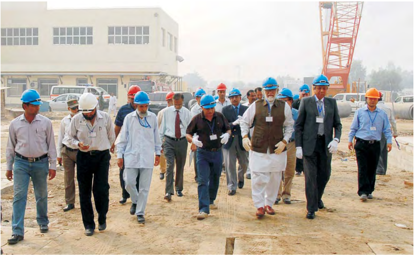
Sardar Aseff Ahmad Ali, Deputy Chairman, Planning Commission and Dr. Samar Mubarakmand, Member (S&T) Planning Commission along with Dr. Ansar Parvez, Chairman, PAEC and other PAEC officials visiting under construction Chashma Nuclear Power Plant (C-2).
