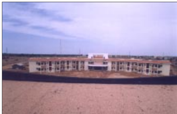
SRI Guest House nearing completion.
