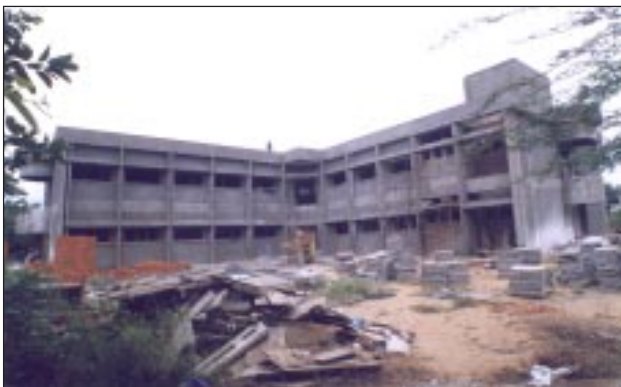
SRI building under construction.
