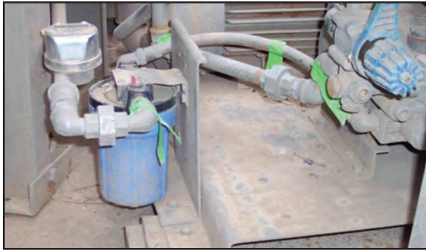
Figure 5. Trailer 1 water filter.
