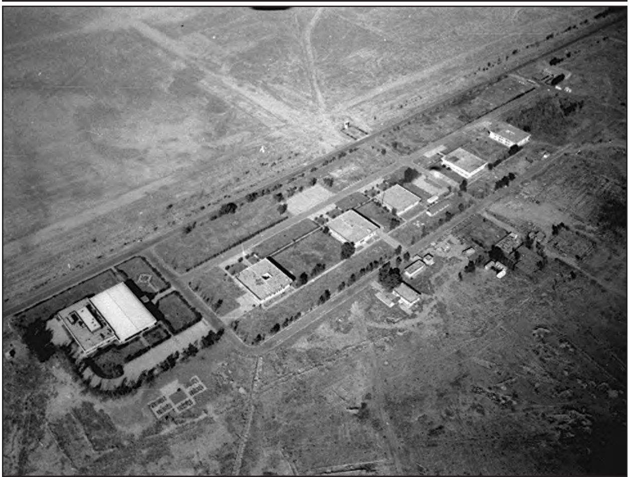
Figure 8. Al Muthanna administration support area razed after 1994.
