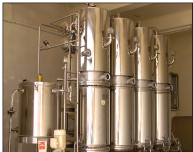
High grade water production plant.
