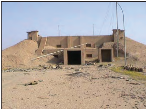
Figure 29. Small bunker with lightning protection.
