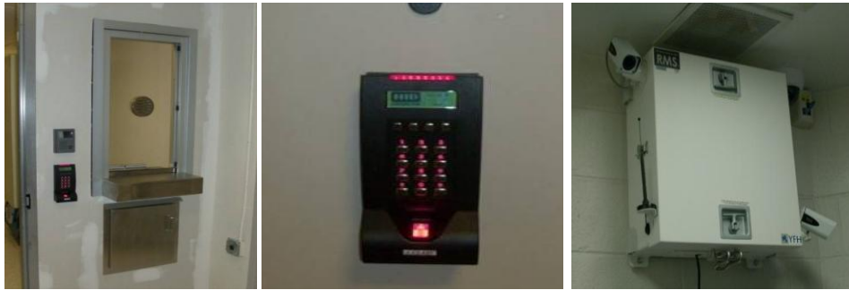
Figure 3. The biometric access control at the bullet proof window entrance of the irradiator and the RMS system provided to Mount Sinai by the US DOE-NNSA-ORS.
